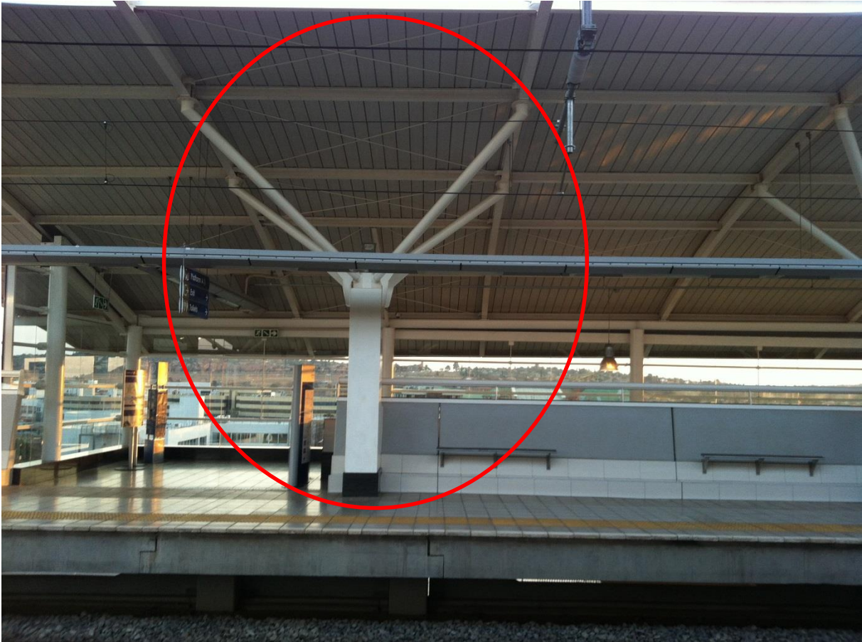
Figure 2: Support columns on the platform
