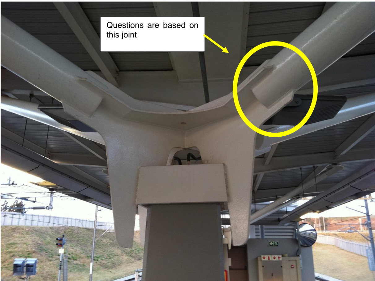
Figure 3: Connection of the steelwork on the concrete column
