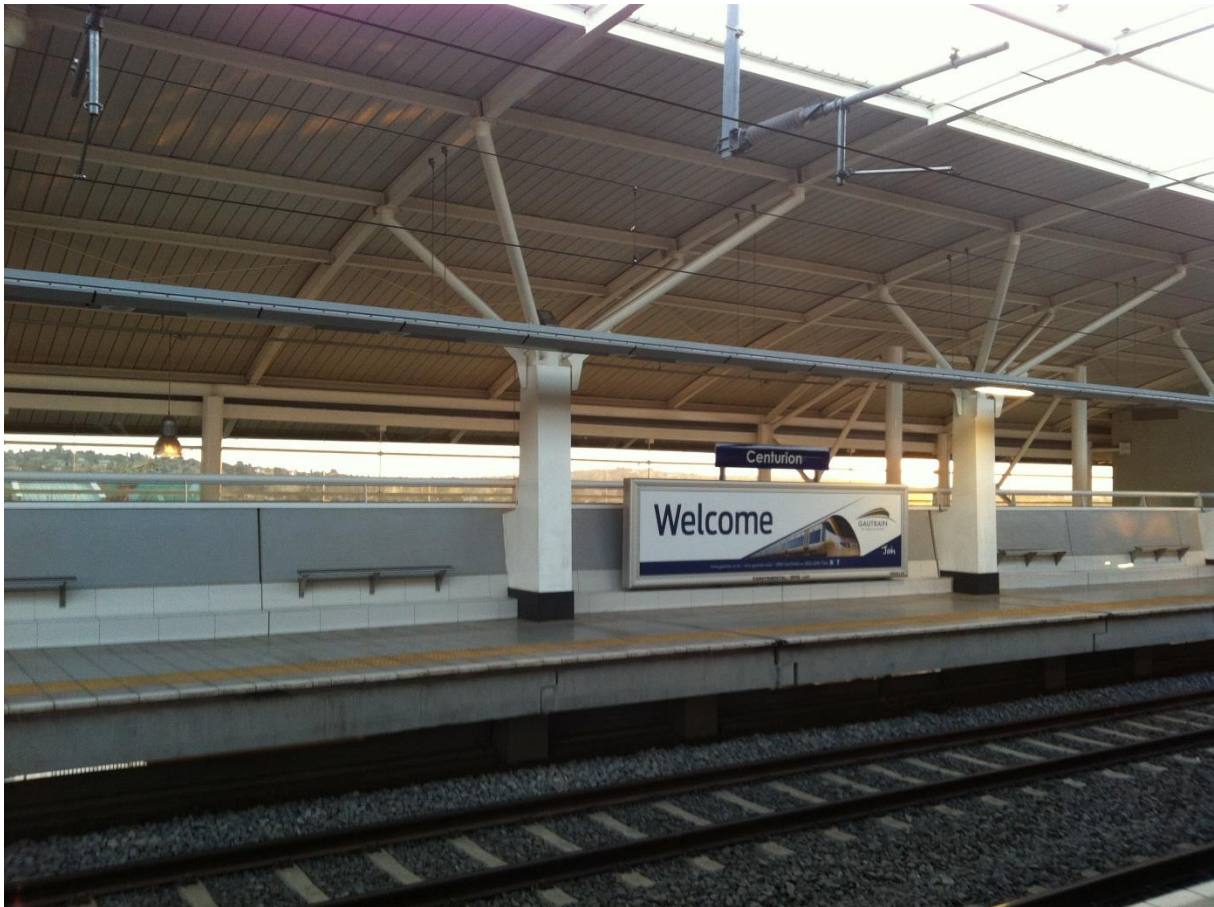
Figure 1: Roof support super structure at the Gautrain Centurion station
